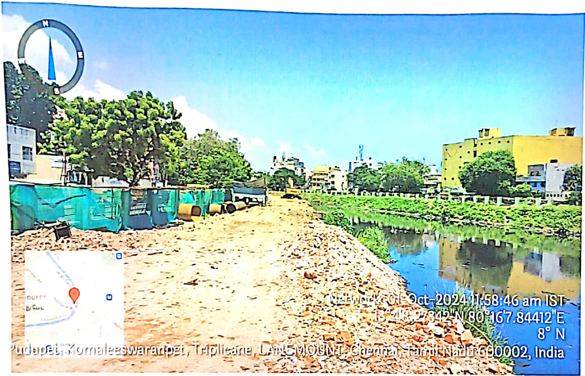
Chinthadripet (near Harris Road bridge)
