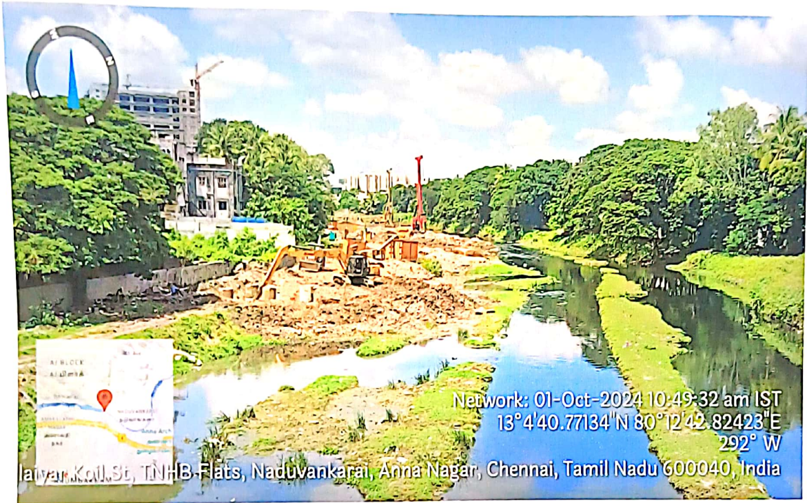
Anna Nagar, Naduvankarai Bridge
