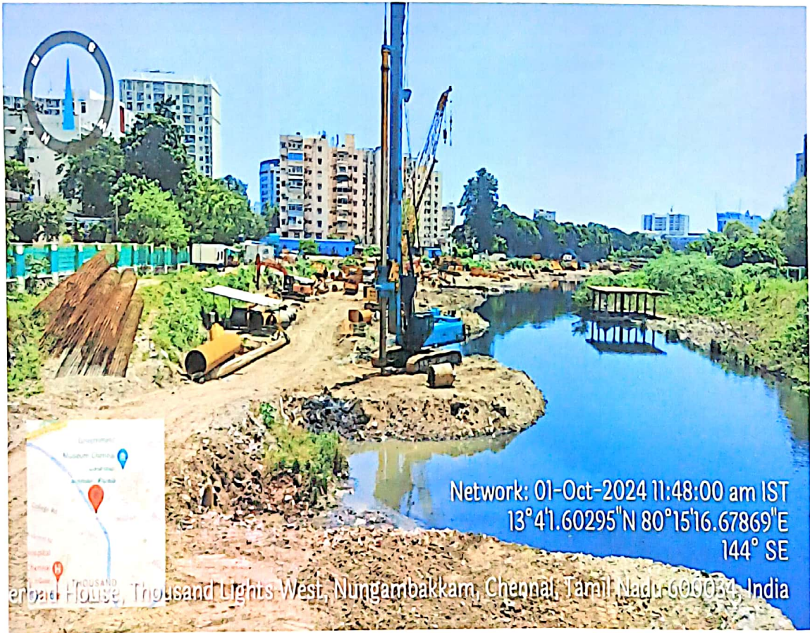
Nungambakkam near College road bridge
