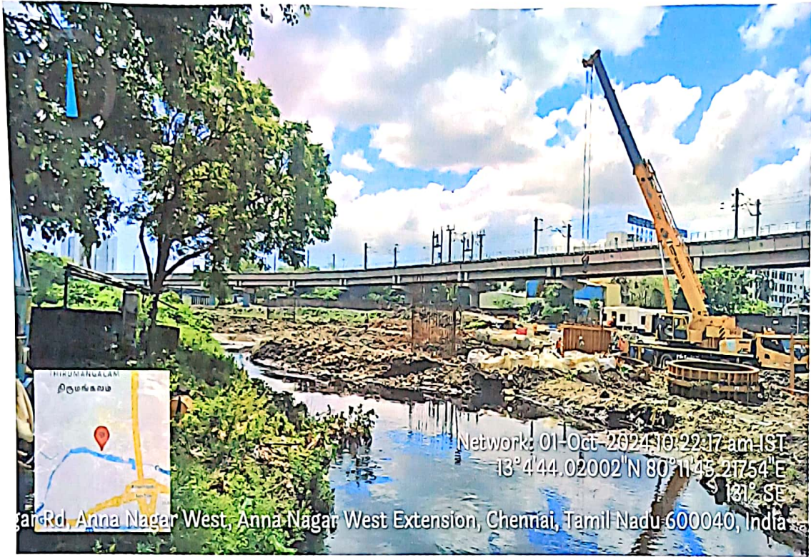
Inner Ring Road Up Stream (Near Sathya Sai Nagar)
