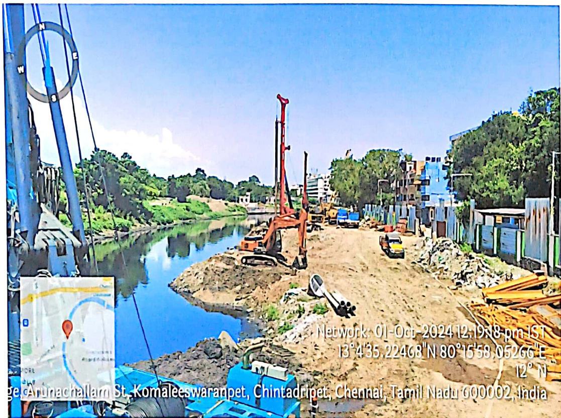
Chinthadripet(near Harris Road bridge)
